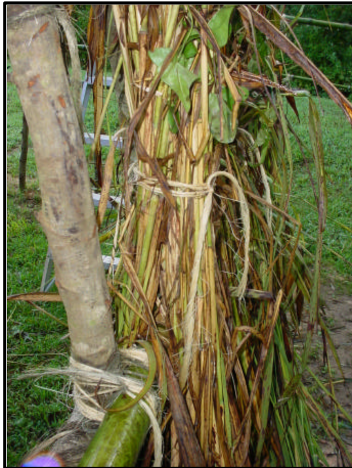
Figure 51. The grass thatching, illustrating how each bundle was hung over the cane stringers. The tied bundles were added from the bottom stringer up to the smoke hole.
