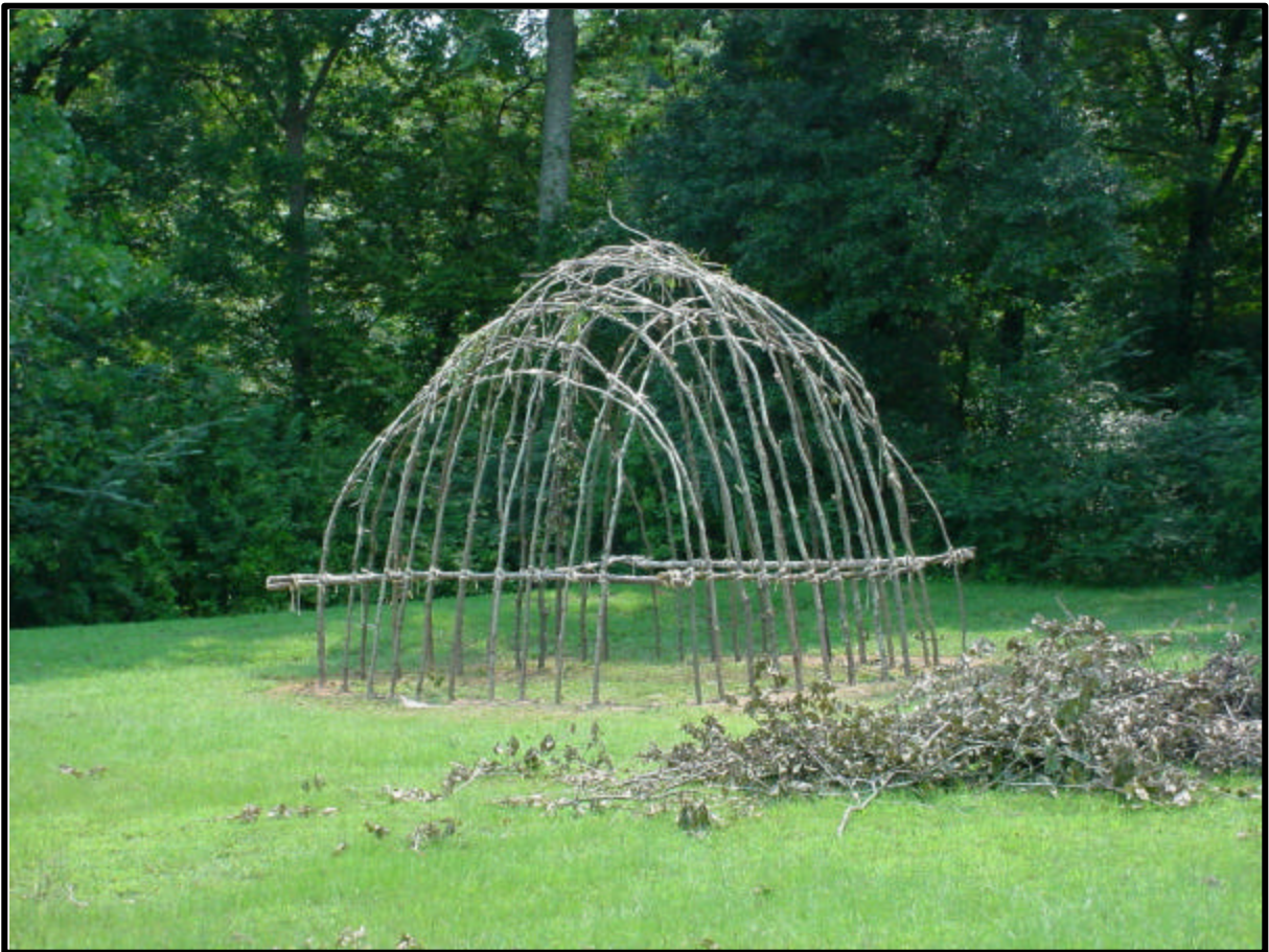
Figure 47. The completed wooden framework of the structure.
