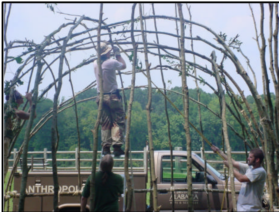
Figure 46. The middle of the bending process. Most of the poles are tied, but the four in the center of the wall in the foreground are still straight.
