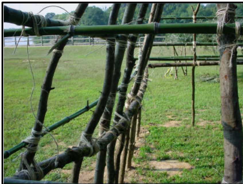
Figure 48. Photograph demonstrating the inward force on the horizontal supports. Note the piece of cane behind the supports which shows the position of the pole before the bending.
