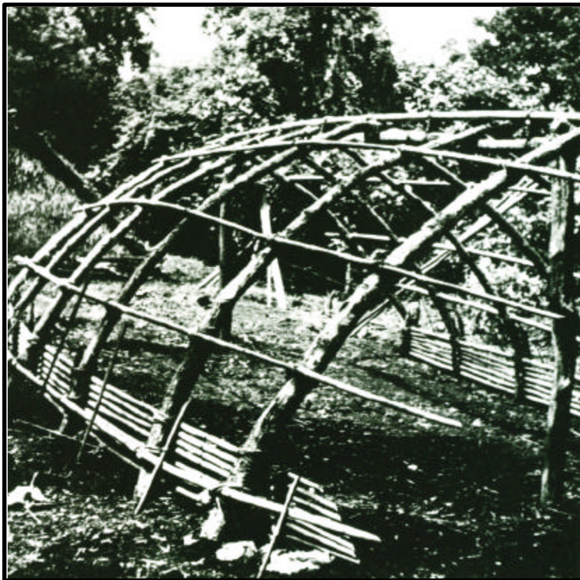
Figure 11. A New Hebridian flexed pole house in Melanesia that possesses two internal roof supports used to hold up a ridge pole in the center of the structure (from Guidoni 1975: 122).
