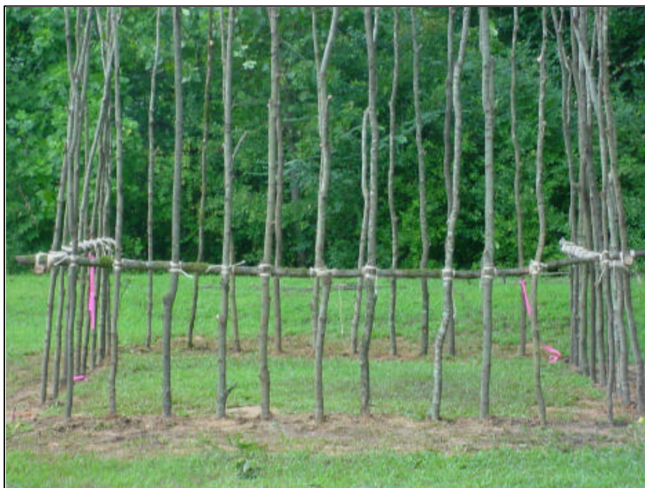
Figure 44. The experimental structure after the addition of the horizontal supports.
