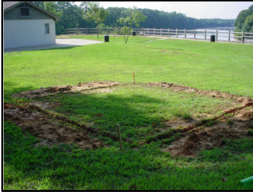
Figure 42. The wall trenches of the experimental structure.
