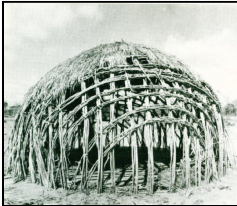
Figure 5. An illustration of Galla house construction in Kenya (Andersen 1977: 36).
