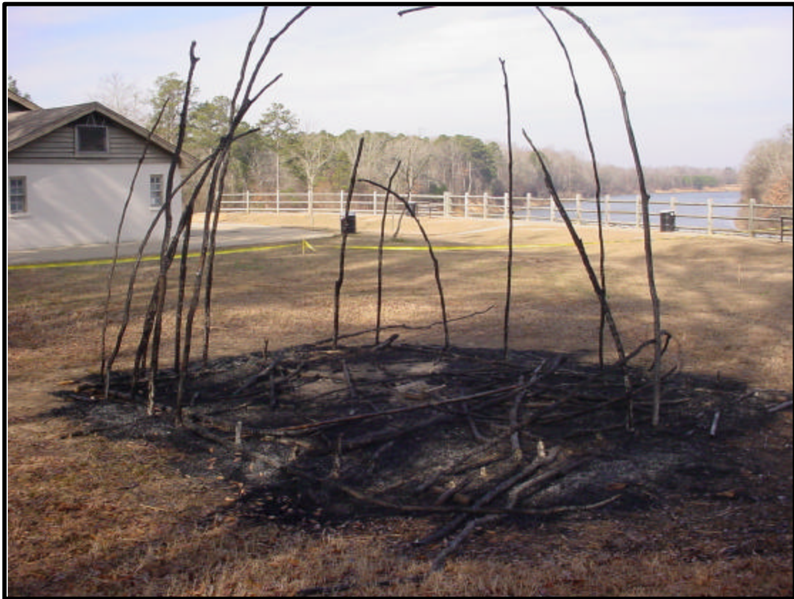
Figure 54. The burnt remains of the house, lying as they fell. Note how most poles were burnt through at the base, but otherwise remain intact.
