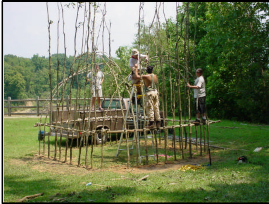
Figure 45. The beginning of the bending process. The poles were bent in sets of two, starting with the outermost poles of each trench and working in towards the center.
