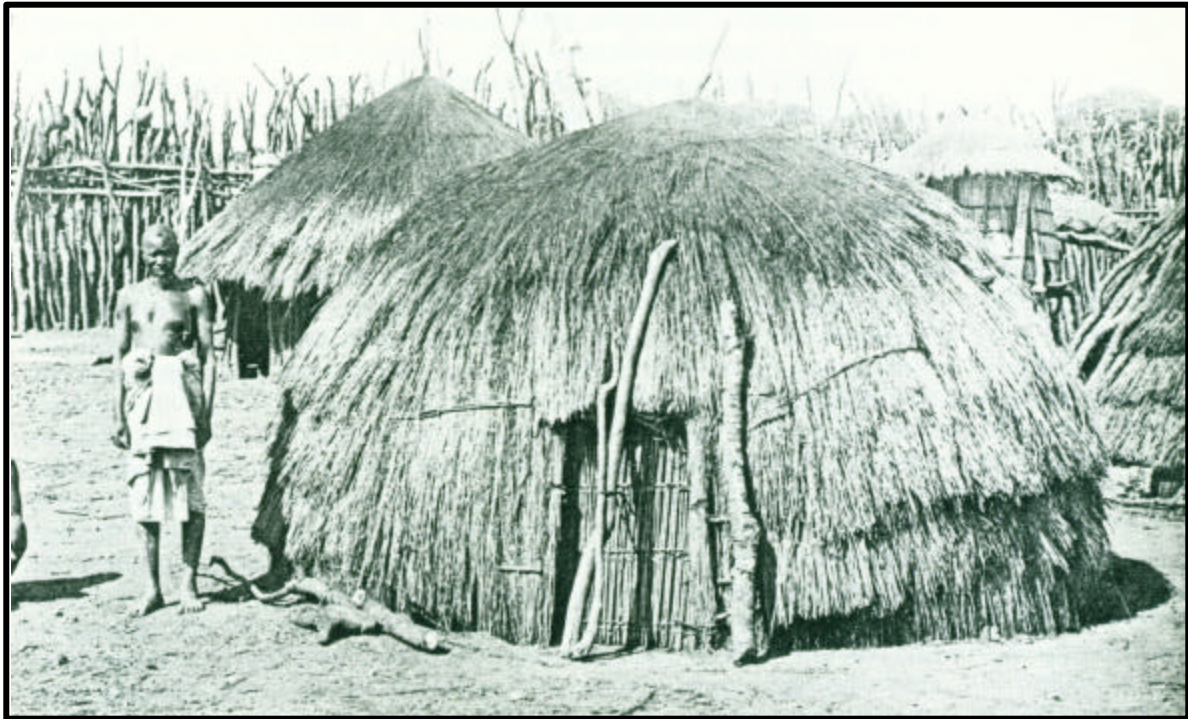
Figure 7. A Nyika flexed pole house in south-western Tanzania around 1900. Notice the rigid post structure in the background (Denyer 1978: 115).
