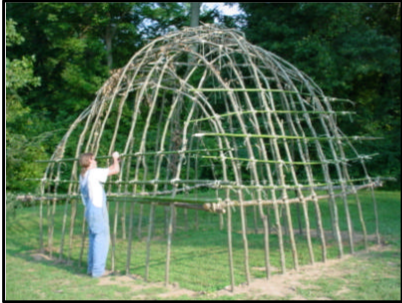
Figure 49. The complete framework with cane horizontal supports tied on. Note how the cane poles are positioned above the horizontal support and continue until the interwoven framework is reached.
